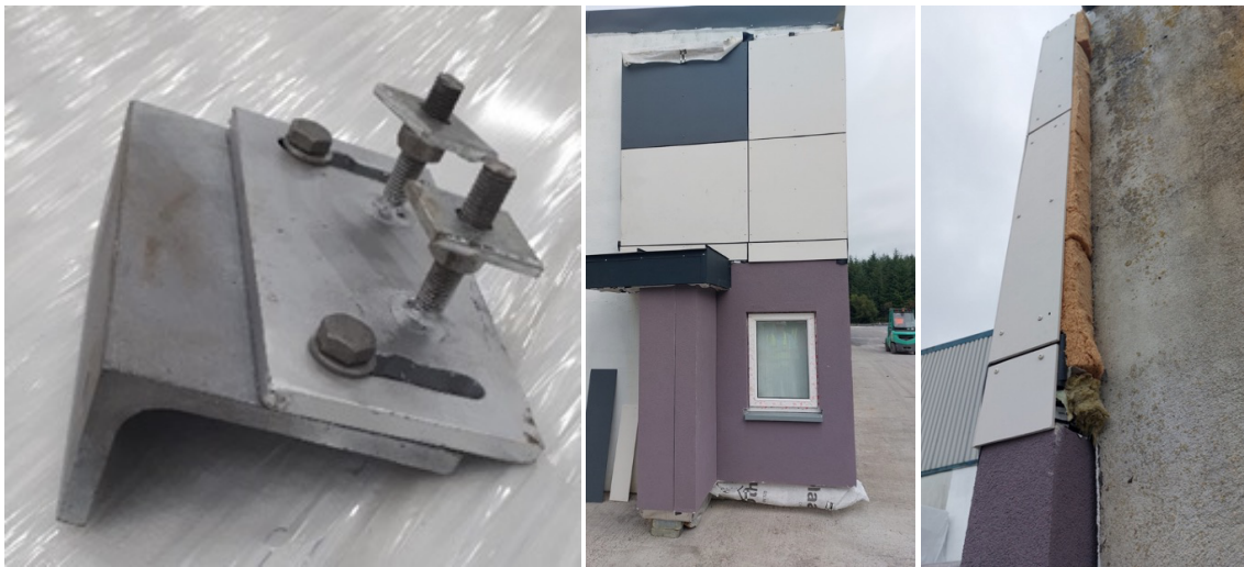
Figure 9 | Mock-up Stage 2 with LHS revised brackets allowing for minor tolerance in three planes, Centre - revised upper panels with new cement board lining and RHS – revised backing insulation
