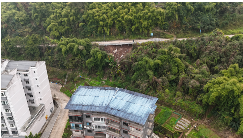
Figure 2 | Full view of the slope site
