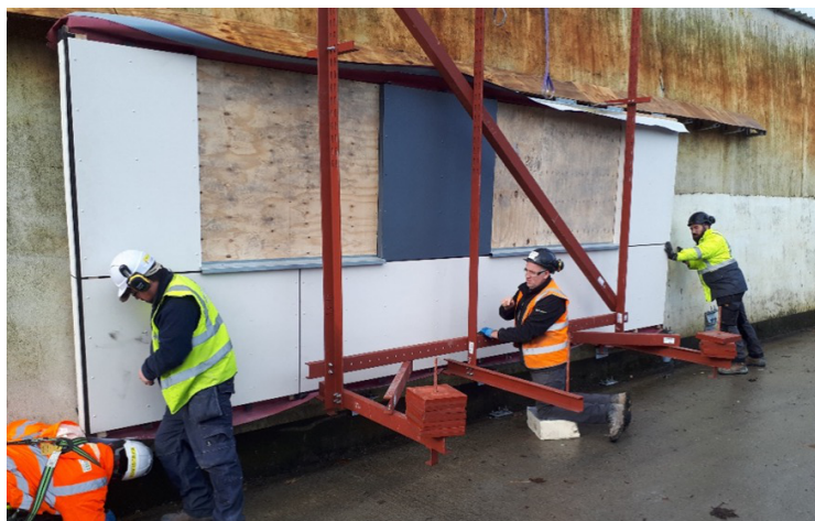
Figure 10 | Showing final mockup full scale panel installation under eaves method being tested
