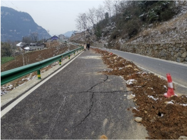
Figure 2 | Road Cracking
