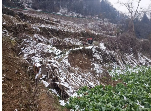
Figure 3 | Local Collapse at Slope Toe
