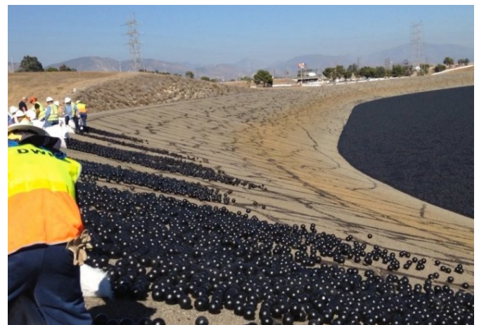
Figure 1 | Deployment of shade balls at the LA Reservoir [7]
